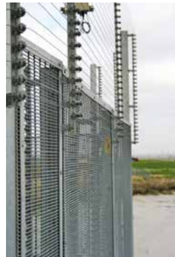
Electric fence topping to mesh fencing
