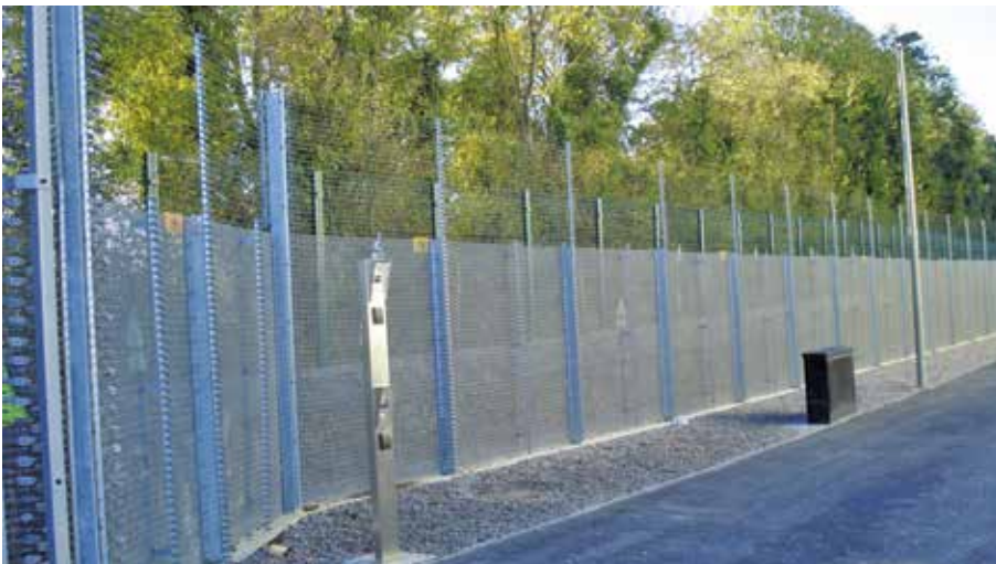
Full height electric fence
